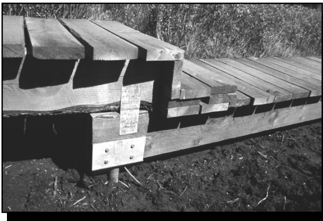
Figure 38—A helical pile was used for this boardwalk. Stringers are attached directly to the beam saddle, helping to keep the boardwalk close to the ground.
