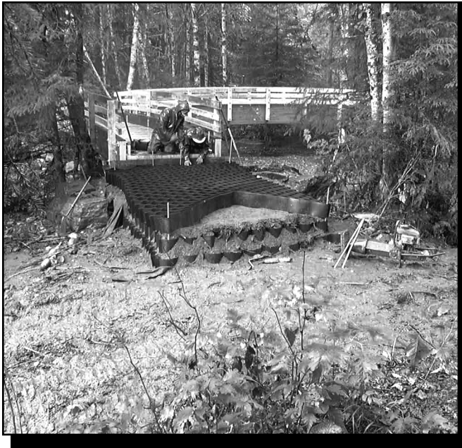
Figure 72—Geocell being laid in courses for a bridge approach. When the approach is completed, the geocell will not be visible.
