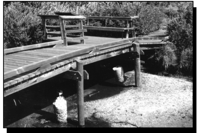
Figure 44—Know your soil conditions. Concrete end-bearing piles settled 1 to 2 feet here and had to be replaced with these log friction piles.
