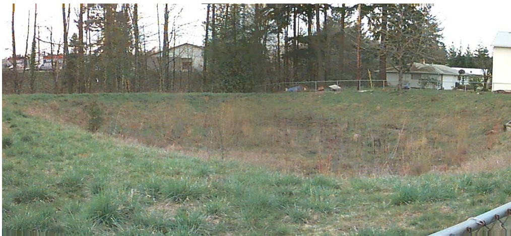
Clean Water Services at corner of S.W. Cornelius Pass Road and W. Baseline Road Collects Storm Water Runoff from Roadside and Roads
