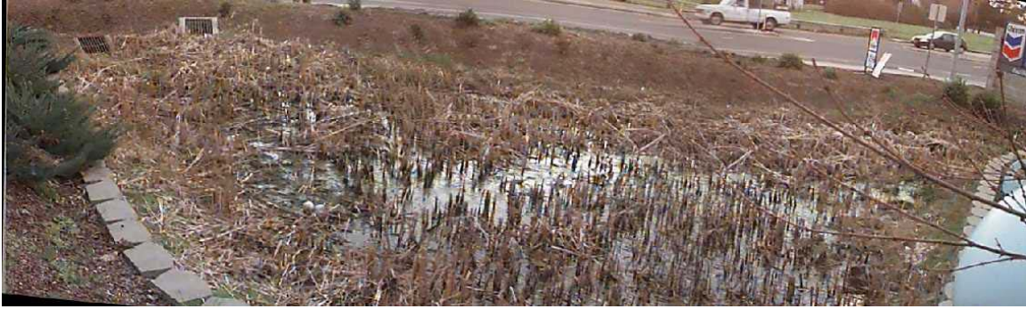
Commercial Pocket Constructed Wetland at the corner of S.W. 185 th Avenue and N.W. Walker Road in Washington County serving the Storm Water Drainage from a Gas Station and an Oil Change Business.
