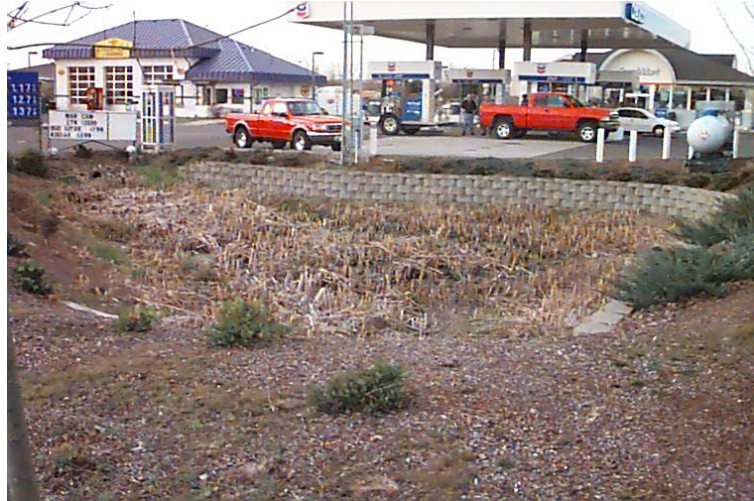
Commercial Pocket Constructed Wetland at the corner of S.W. 185 th Avenue and N.W. Walker Road in Washington County serving the Storm Water Drainage from a Gas Station and an Oil Change Business.
