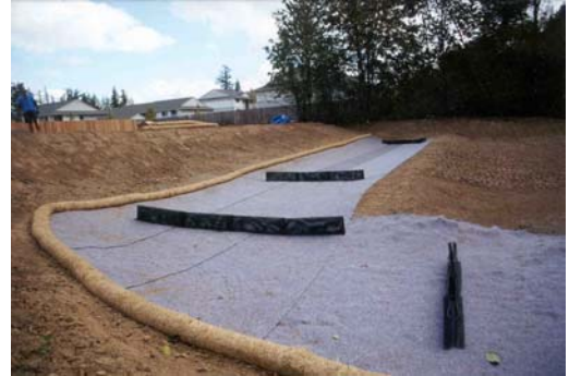
Swale with erosion/turbidity protection blanket and Check Dams installed.
