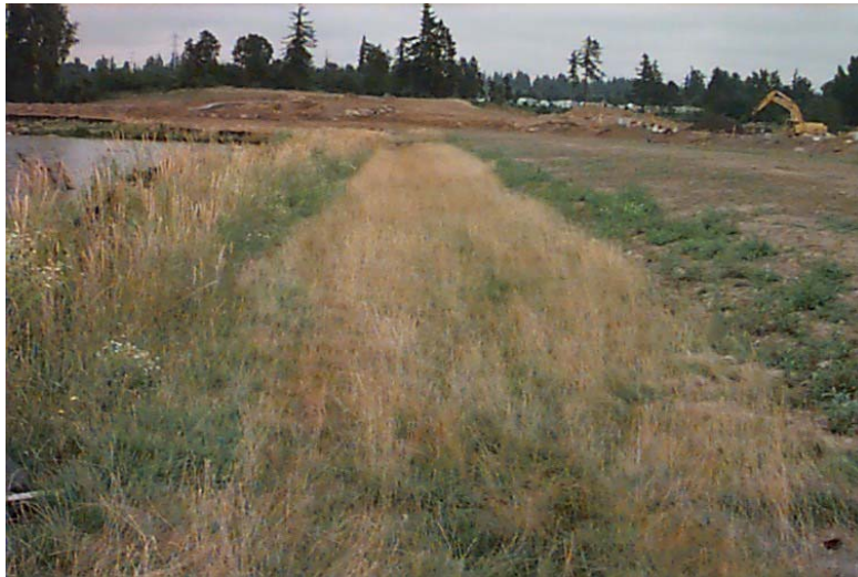
Residential Development Grassy Bioswale at Fairview Lake used during subdivision construction
