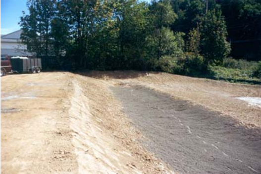
Swale with ceramic grit installed.
