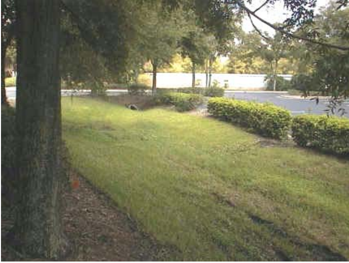
Lawn Bioswale in Texas
