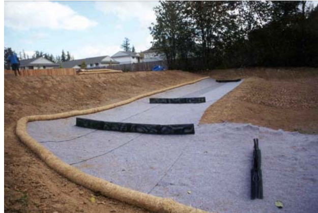
Bioswale System Liner
