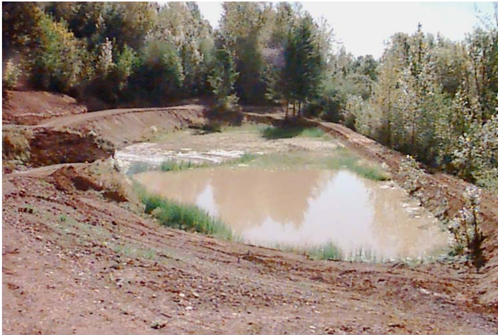
Initially a Sediment Pond Off Judd Road in Clackamas County
