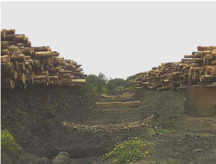
Construction of bioswale in 2001 (Notice swale divider in picture on the right)
