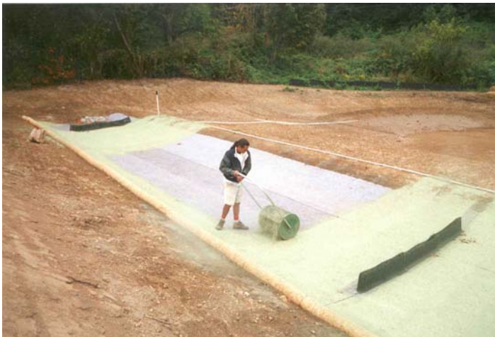
Swale with seed/mulch being applied on top.
