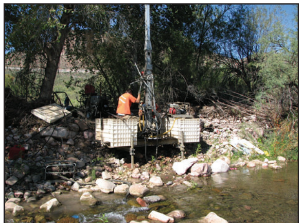
Figure 4-5. Hand augers can be used to bore holes for installing a groundwater monitoring well. Mounted power augers may be used in cobble or hardpan substrate.
