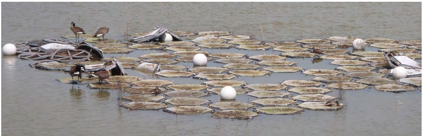
FIGURE 12. Jannock Pond FTW pilot project, Mississauga, Ontario after 100-year storm event. Multiple modules were flipped but module-module tethering system and anchor lines were all intact.
