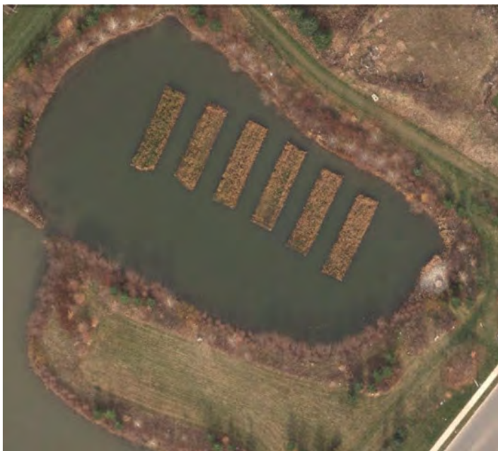
FIGURE 2. Pond 10 Thermal Mitigation FTW, Brampton, Ontario (Fall 2011, 1 year post installation).
