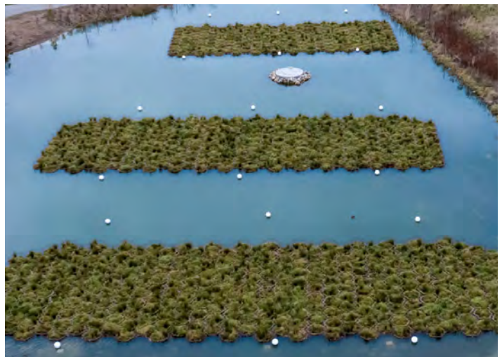
FIGURE 14. PhytoLinks FTW installation Brampton, Ontario Canada (2017) showing 6 anchor lines (white buoys) per grouping of modules.
