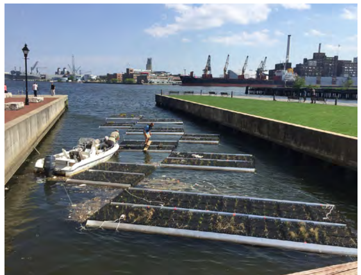
FIGURE 5. Bond Street project- original orientation (Spring 2017).
