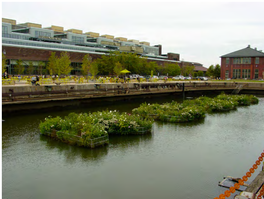
FIGURE 1. BioHavens are part of an industrial waterfront beautification project at the Urban Institute in Washington, DC. (Note: All photos for this article provided courtesy of Floating Island International, Inc. – permission granted March 22, 2019.)
