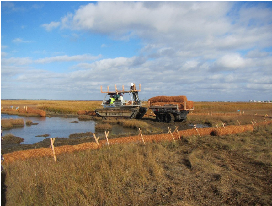
FIGURE 2. Site preparation prior to thin layer sediment application included placement of coir logs to target areas receiving sediment additions (top). Thin layer placement of dredged materials involves spraying a dredged sediment slurry onto the marsh surface (bottom). (Photo courtesy of Tim Welp)
