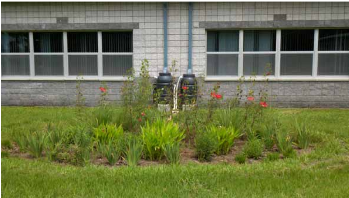
Figure 1: Rain garden at Kanapaha Middle School, Gainesville, Florida.
